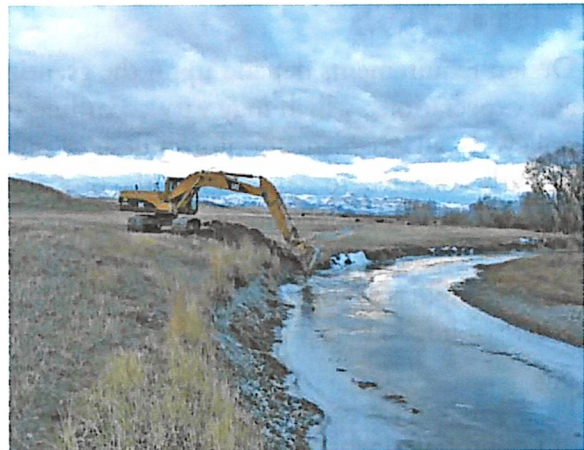
Construction activities on the bed and banks of perennial streams generally require both state and federal permits. No floodplain permit was required for this project.
