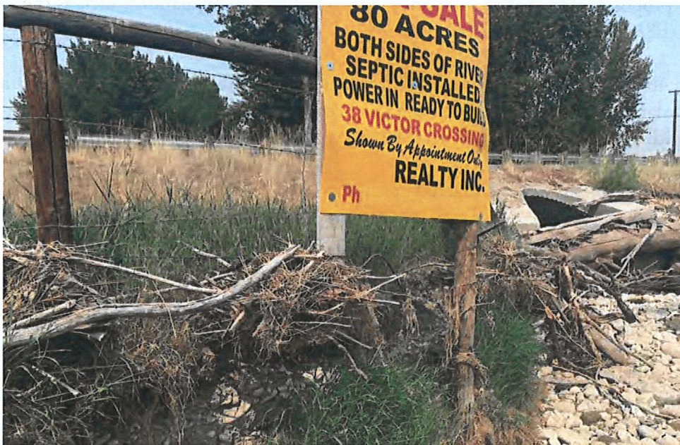
Although floodplain permitting can be time consuming and costly, the process helps ensure that existing and future development minimizes risk of flooding problems. Note the high water mark/debris at the base of the sign.
