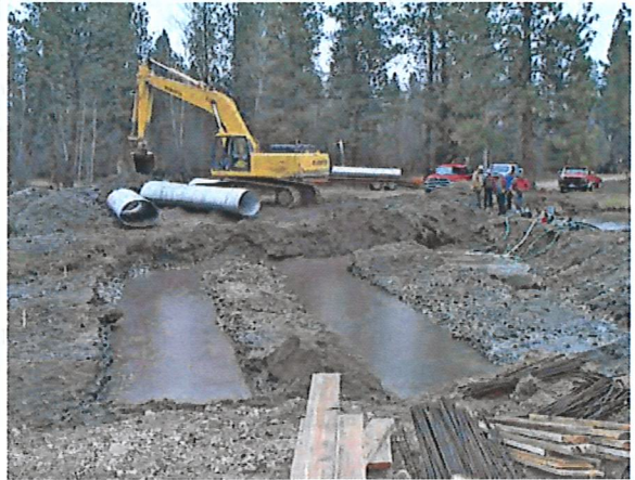
Dewatering construction areas with pumps requires a MPDES permit when discharging to State waters.
