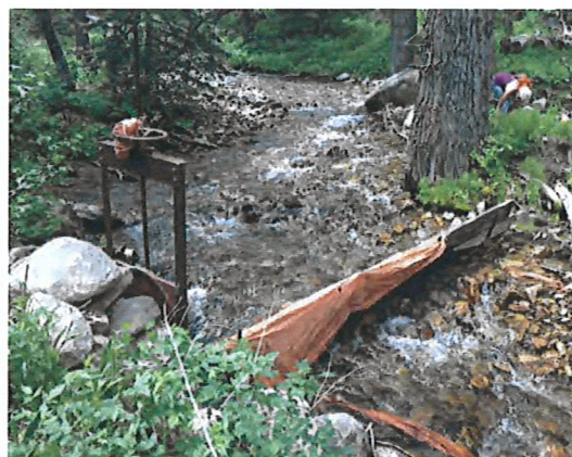
Replacement or maintenance of irrigation structures are common 310 projects.
