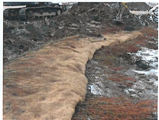
Cuttings should be trimmed so approximately one-third of the stem is exposed.
