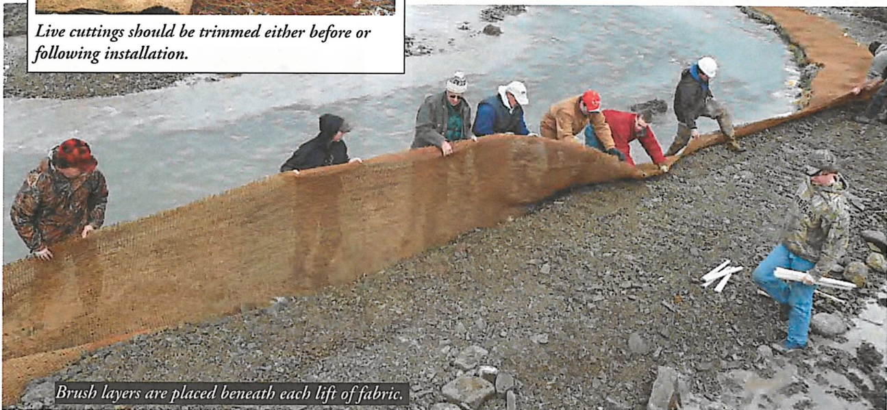
Brush layers have the best survival when placed near the water table or in moist soils. Irrigation may be required in droughty or coarse soils.
