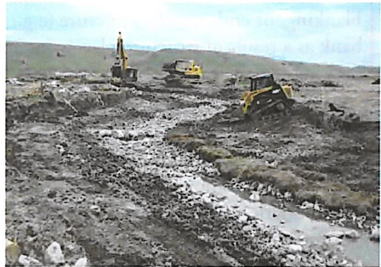
Ideally, in stream work can be completed “in the dry” by diverting or pumping water around the site.
