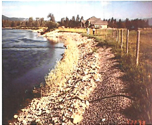
Live willow cuttings seem to survive best when cut and planted in the early spring prior to bud break.
