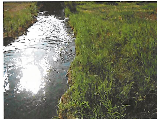
Restored streambank using coir fabric, willow plantings and sod (same location as above photo).
