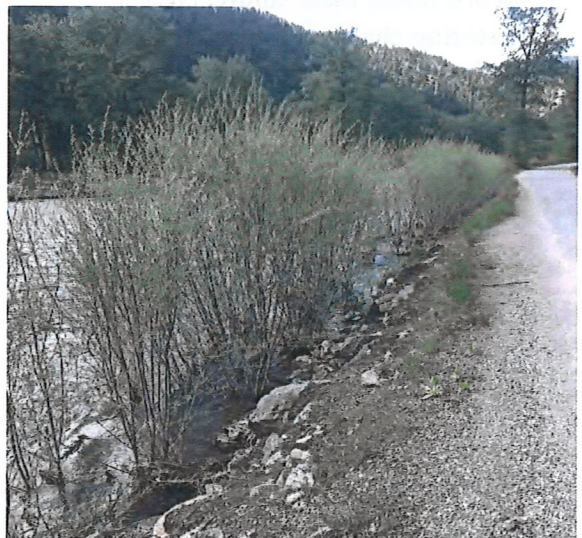
Willow can be successfully incorporated into rip-rap providing added water quality and habitat benefit.
