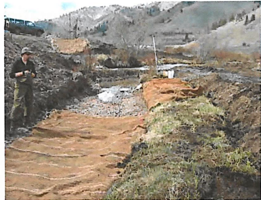
Restoration of streambanks using bioengineering techniques can provide excellent bank stability and promote natural channel function.
