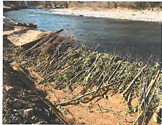
A mix of live and dead brush provides bank roughness and revegetation. A high density of stems (10-15 per foot) is common.
