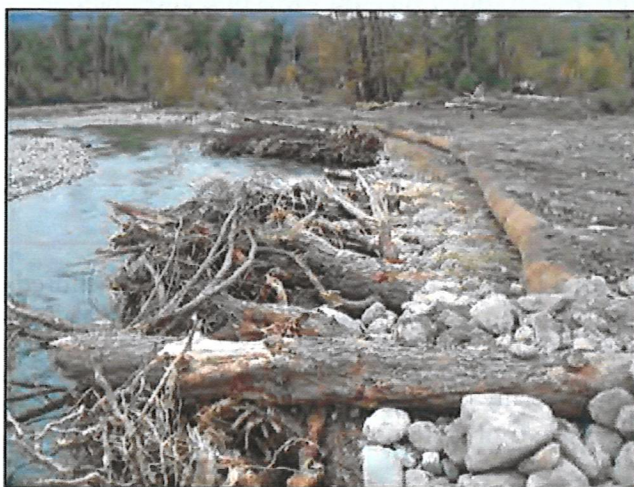
Example of a constructed large wood structure type 1
