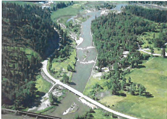
These large weirs eventually failed because they were built too high, and restricted sediment passage. Removal of these structures came at a high cost.
