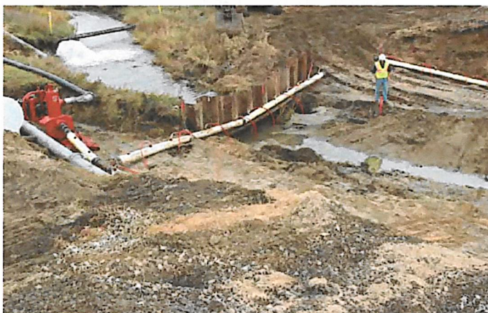
Pumping water around a construction site is generally feasible only on smaller projects and smaller flow rates.
