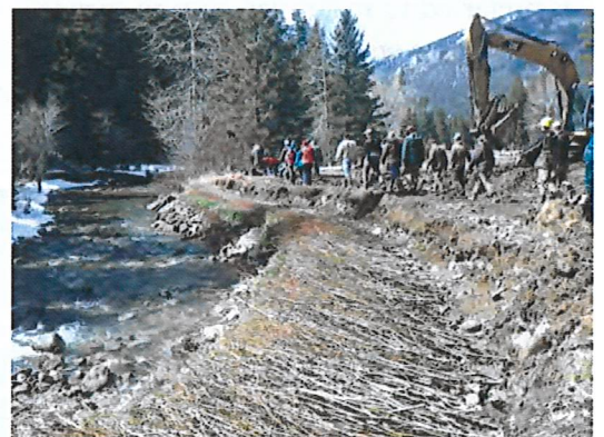
Live brush layers can be used to form a toe where scour depths are not expected to undermine the treatment.
