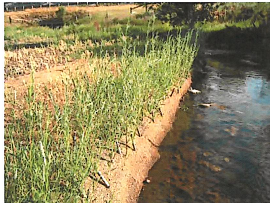
Willow cuttings work well planted through geotextile fabric if the basal end of the cutting can reach the water table. Irrigation is also useful to help establish new cuttings.
