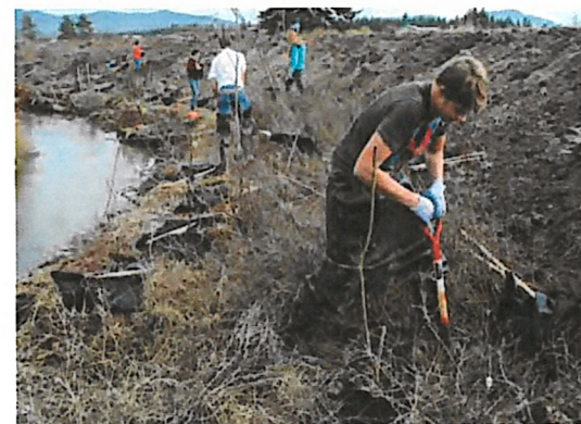
Willow stakes can be planted through fabric or into soils or sod.
