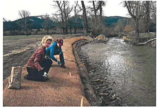
Soil lifts are commonly installed as a single or double layer ranging in thickness from 1 to 2 feet in depth.
