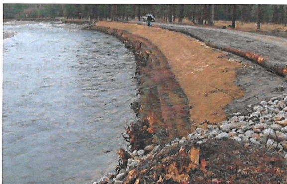
Encapsulated soil lifts with LWD toe and willow cuttings.
