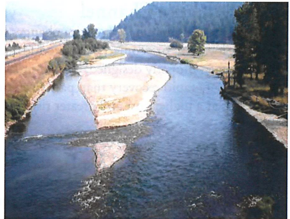
Rip-rap on channelized reaches will limit the ability of the stream to re-establish equilibrium.
