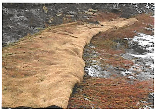
Live cuttings should be trimmed either before or following installation.
