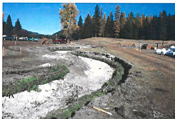
In moderate scour or erosion applications, toe protection can include brush layers, fascines, and small woody debris.
