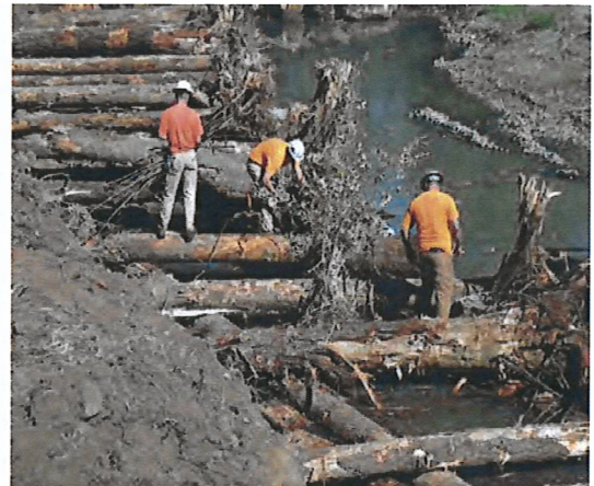
Placement of large woody debris forms the foundation of many stream projects on large rivers.
