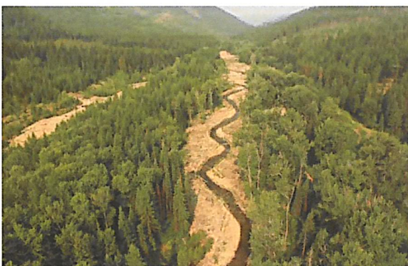
Re-establishing meanders in a channelized reach requires substantial hydrology and engineering design expertise.
