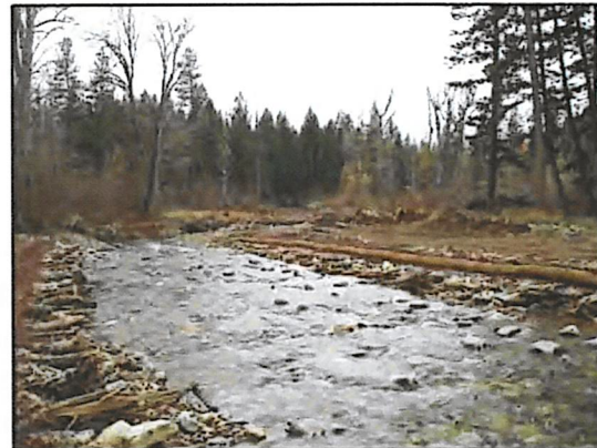
Example of a constructed vegetated soil lift type 1
