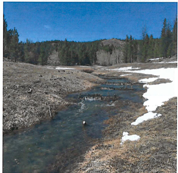
Recently installed BDAs slowing runoff and aggrading an incised channel
