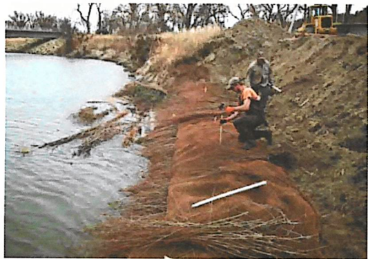
Brush layers have the best survival when placed near the water table or in moist soils. Irrigation may be required in droughty or coarse soils.
