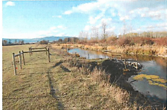
Riparian fencing will allow woody vegetation to re-establish and a water gap provides controlled access to water for livestock. Larger riparian enclosures can compliment rotational grazing and provide additional room for streams to migrate.
