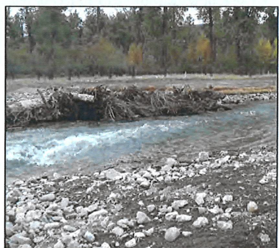
Example of a constructed large wood structure type 1
