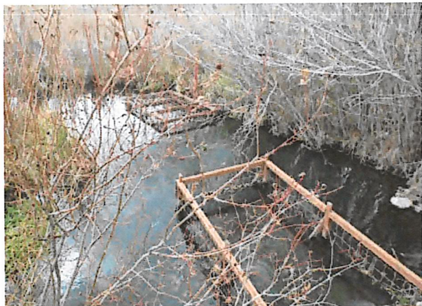
Beaver deceiver™ installed at upstream end of culvert to prevent beaver from damming.
