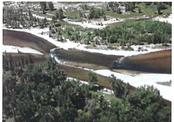
Large weirs on unstable rivers can run to over $100,000 and still carry substantial risk of failure. Bedload deposition and scour can result in channel changes that bury weirs and scour away footings. Rivers may quickly cut new channels around the structure.
