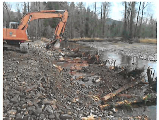
Large woody debris foundations are typically backfilled with some amount of large rock and native fill for ballast.
