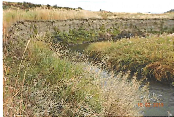
Before - An eroding bank (e.g., terrace or hillside) can sometimes be stabilized by construction of a bankfull bench. This may require channel reshaping to offset fill placed during construction of the bench.
