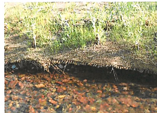
Biodegradable geotextiles can last 2 to 4 years while vegetation becomes established. Note, however, that the fabric in this photo has been abraded in the first year. Ultimately, all biodegradable fabric treatments rely on vegetation for long-term stability.
