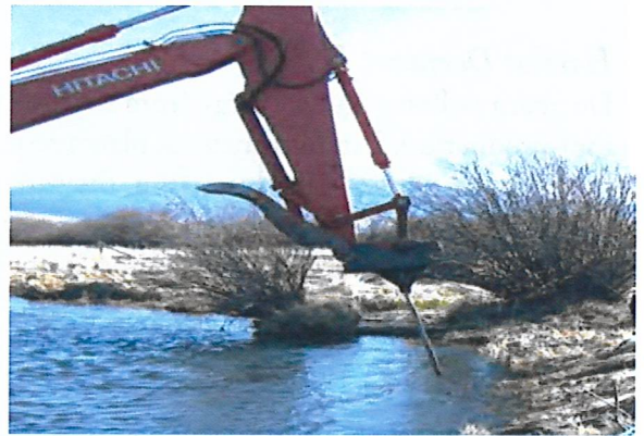
An excavator with a dibble is used to place plantings.
