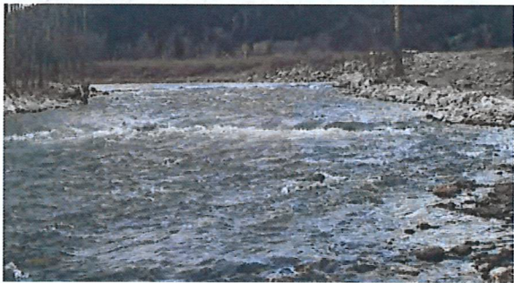
Large weirs must frequently be built in series to avoid large drops exceeding structural stability. Construction of weirs in high bedload transport streams always carries some risk of failure.
