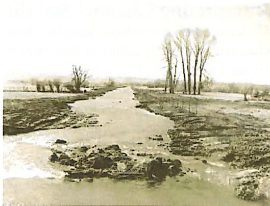
Channelization of streams frequently results in incised channels in disconnected floodplains. Big Spring Creek near Lewistown was channelized at the turn of the century.
