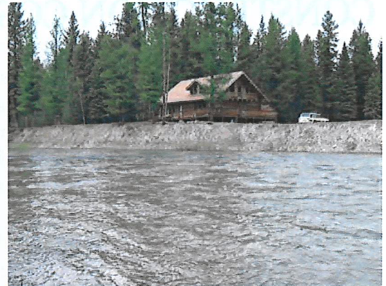
Homes built on river terraces may be out of the floodplain but at risk from river migration. Protecting these sites can be costly and technically challenging.
