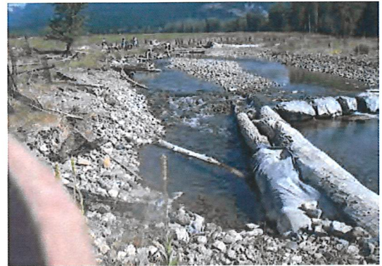
Any instream structures, including habitat features, require careful design and placement to be successful. Channel scour and fill can result in structure failures.
