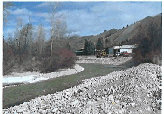
Gravel excavation in aggrading channels seldom results in satisfactory solutions to flooding.
