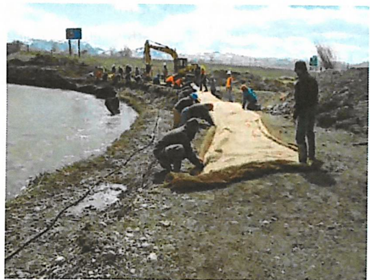
Bioengineering treatments can be labor intensive, especially for installation of fabric. Bioengineering is preferred where vegetation treatments can be successfully established.
