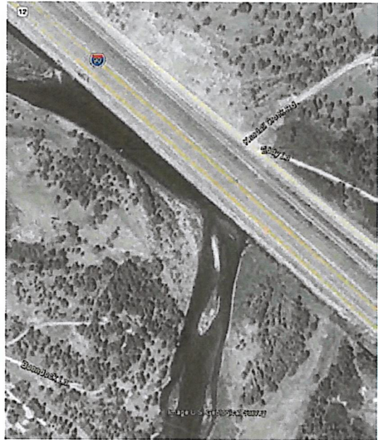
Physical constraints (highway above) may limit restoration options. (Clark Fork, 1995)
