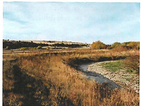
Terrace with brush layer toe and geotextile fabric bankfull bench. This project failed after three years and returned to a similar condition as pre-construction.
