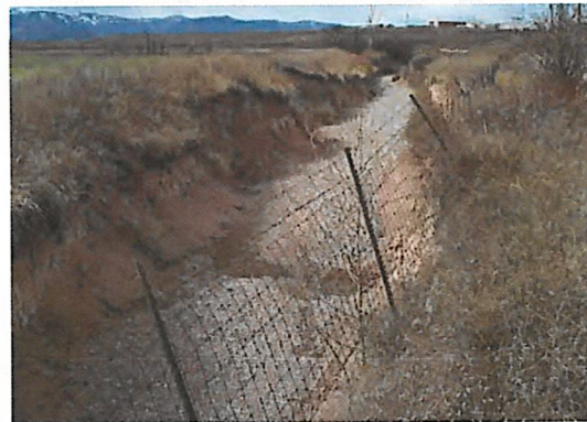
Degrading (scouring/downcutting) channels are common when streams have been straightened.
