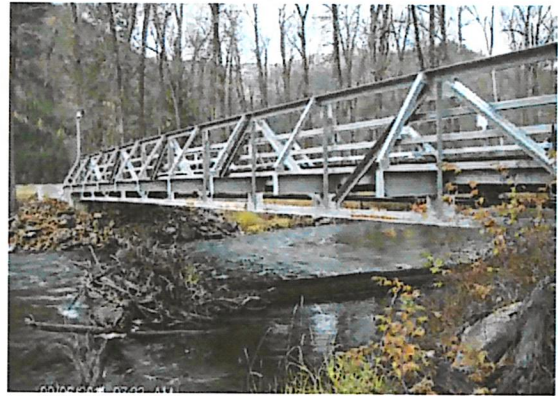
This well-designed bridge has adequate clearance for ice, debris, and peak flows. Note, however, that the abutments do encroach on the channel somewhat.
