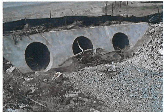
Multiple pipes are sometimes acceptable, but they can catch debris. Consider aluminum box or squash pipes.
