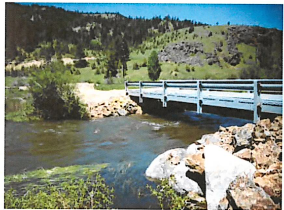
The structural beam on many railcars hangs low and ends up falling below bankfull elevation, which presents risks during high flows.
