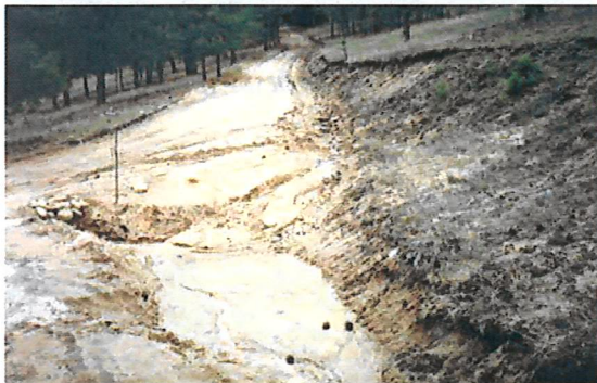
Poor drainage on granitic soils can deliver large amounts of sediment to streams.
