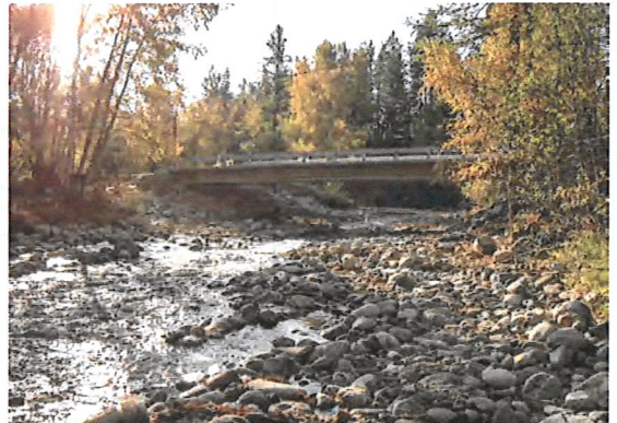
A well designed bridge spans the bankfull channel width (or more) and allows sufficient clearance for passage of flood, ice, and debris.
