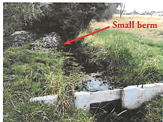
Small temporary berms may be appropriate in some locations as a low-impact alternative to permanent structures.
