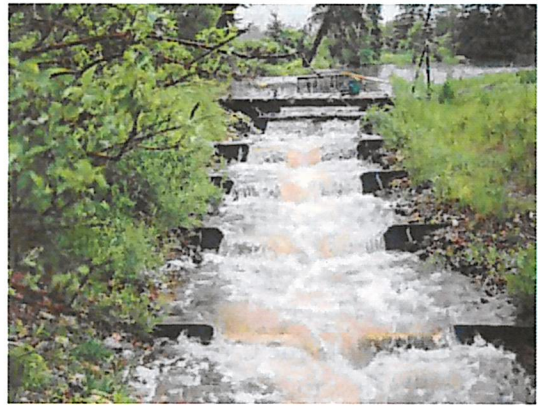
Pool and weir structures can be made of natural materials or engineered structures.
