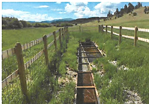
Farmers screens operate with no moving parts and provide good fish protection characteristics.
