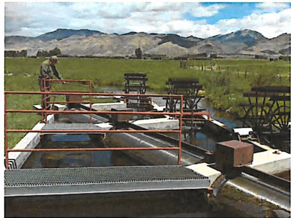
Drum screens can be configured with multiple bays to accommodate a wide range of flows.
