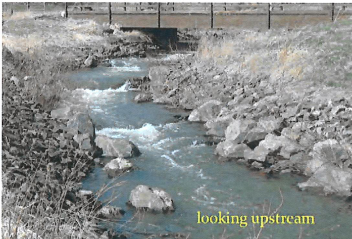
Roughened bypass channel with rock weirs.
