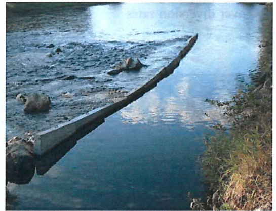
Blocks can reduce the need for streambed disturbance associated with gravel berms. Blocks should be removed following irrigation season.
