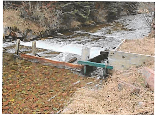
Original stopboard structure and Denil ladder did not provide adequate fish passage.
