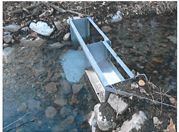
In a Coanda, water flows down and out of a pipe, while fish and debris pass over the screen.
