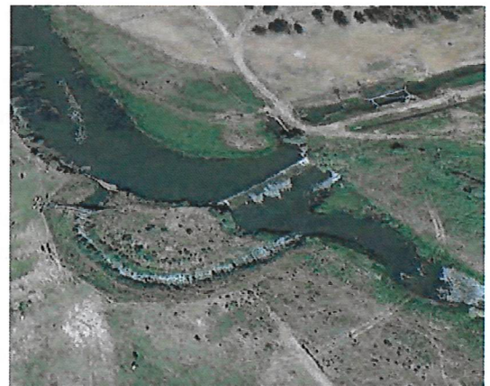
Engineered riffle bypass provides fish passage.
