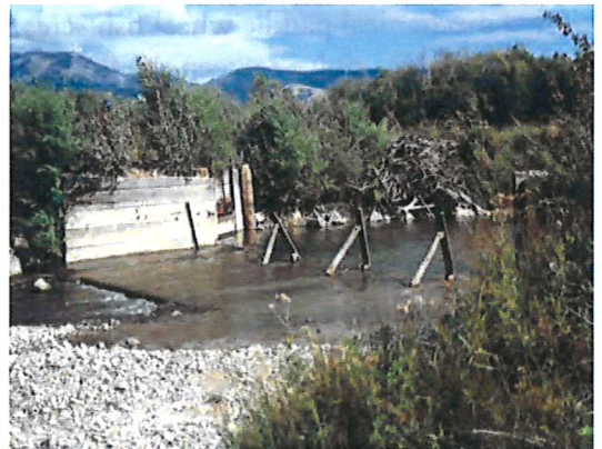
Wooden diversion structures have a limited life but are easily constructed. These type of diversions often form fish barriers because of the stopboards and flat floor.
