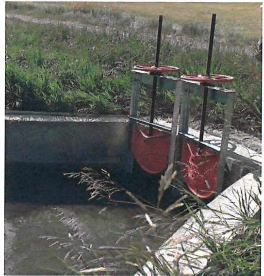
A C-10 gate generally benefits from a headwall to stabilize fill. Rock can work, but the slope leaves the gate frame exposed to ice and debris.
